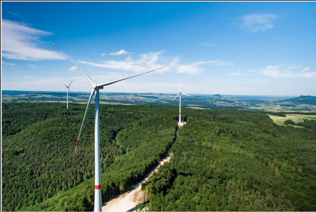
Abb. 6: Fertiger Windpark Verenafohren (Quelle: Jens Scherer, DesignConnection).
